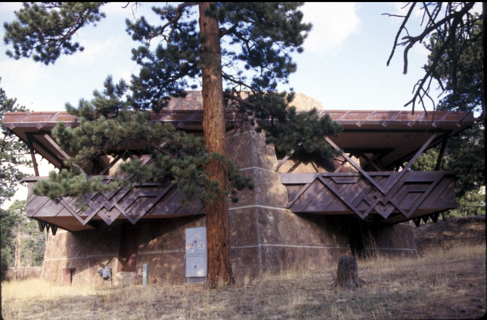
Beaver Meadows Visitor Center, Rocky Mountain National Park, Colorado, Taliesen Associates
